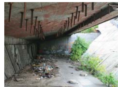
The underground level of “1300 Years Bulgaria”, Sofia, May 2008.
